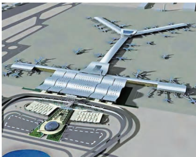
NEW DOHA INTERNATIONAL AIRPORT
